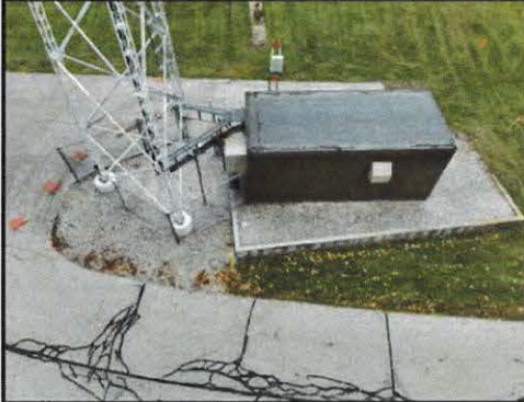
B COMPOUND OVERVIEW
