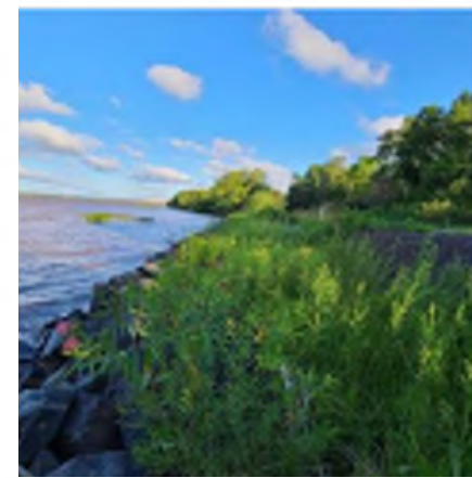
Record-high Lake Superior water levels causing erosion on Wisconsin Point in Superior
