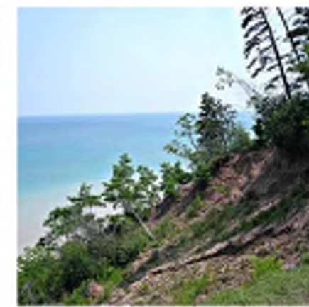
Bluff erosion in Ozaukee County
