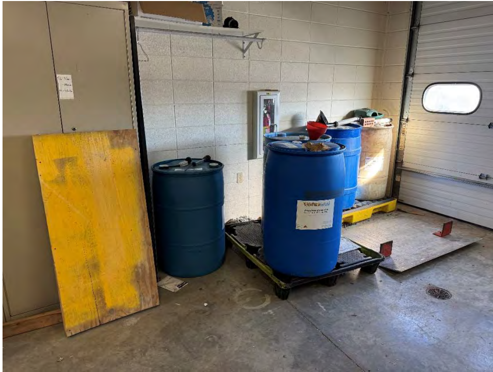
View of used antifreeze storage in the Field House's loading dock area.
