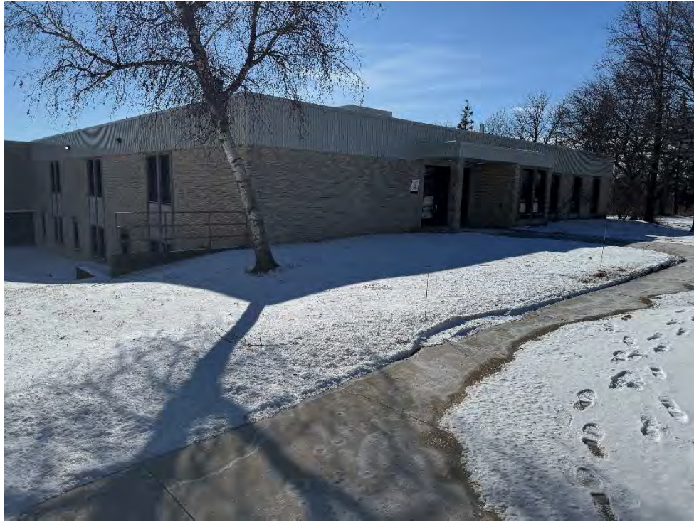
View of the rear of Southview Hall, facing southeast.
