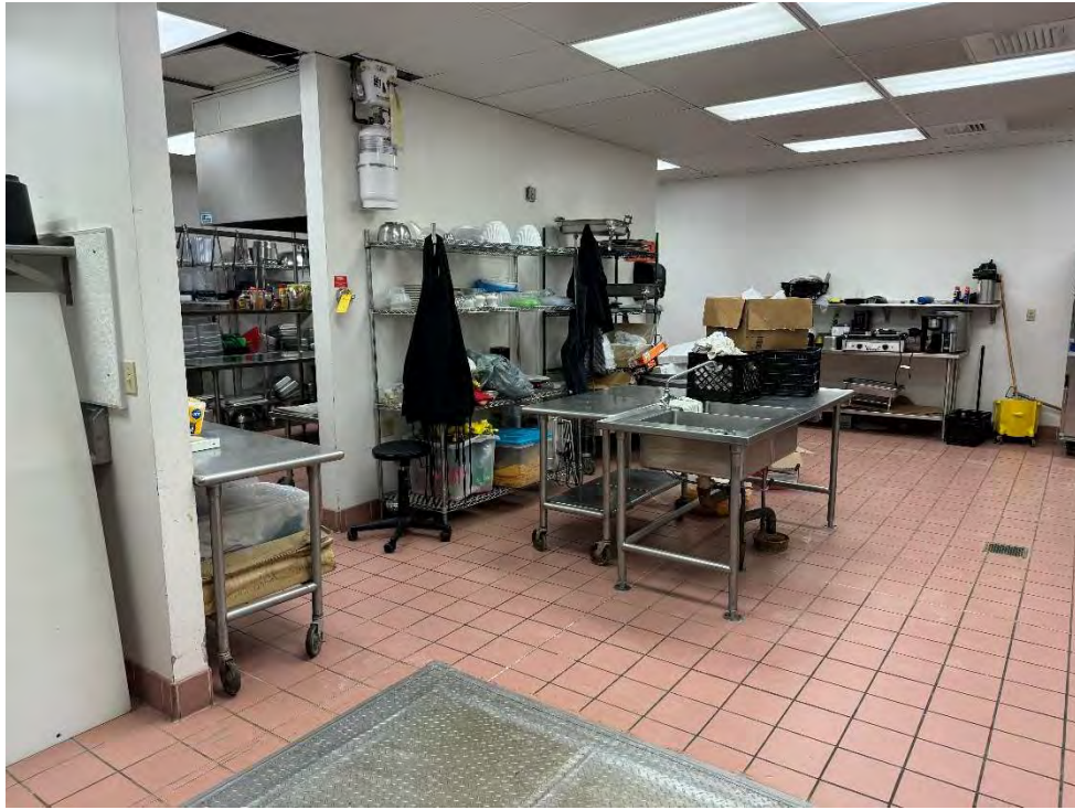
View of the kitchen in Westview Hall. The facility's grease trap is in the foreground.
