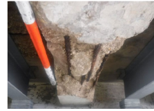
Figure 4.6 Steel Reinforcement Corrosion Causing Concrete Damage
